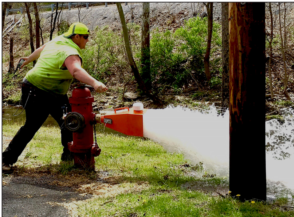
Borough Public Works crew member Tom Feldman works to flush a fire hydrant along Ann Street. Flushing was done to clean sediment from the water system as part of efforts to empty the Borough reservoir for inspection. The orange diffuser holds tablets to neutralize the chlorine in the Borough's drinking water before it flows back into local streams.
