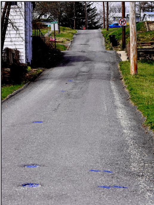
**Blue paint on Chestnut Street marks the location of current pipes to assist the engineers planning the replacement of that key water main.**
