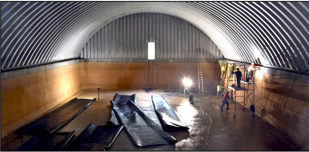
Crews work to prepare the Borough's reservoir for the installation of a liner to stop water leaks.
